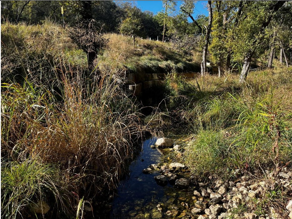
Photo 16. Established vegetation and stabilized infrastructure (bank stabilization #4). Photo taken on 11/21/2024.
