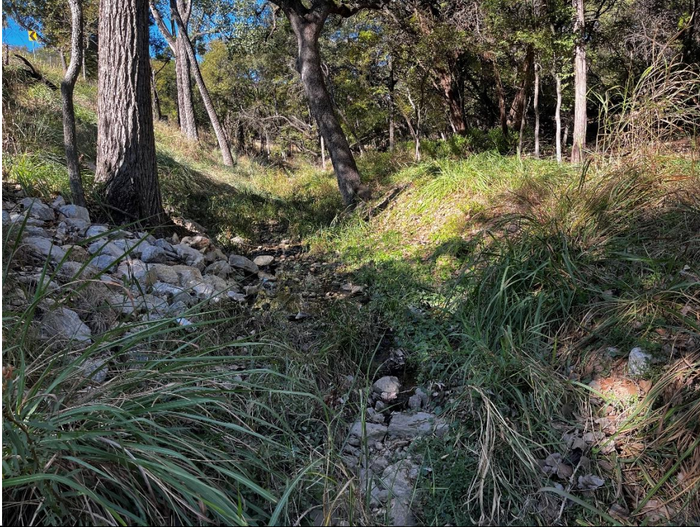
Photo 5. Station 5, between grade control structure #3 and bank stabilization #5, facing upstream. Photo taken 11/21/2024.
