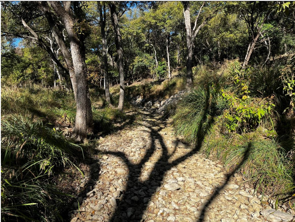
Photo 4. Station 4, between bank stabilization # 2 and #3, facing, facing upstream. Photo taken 11/21/2024.
