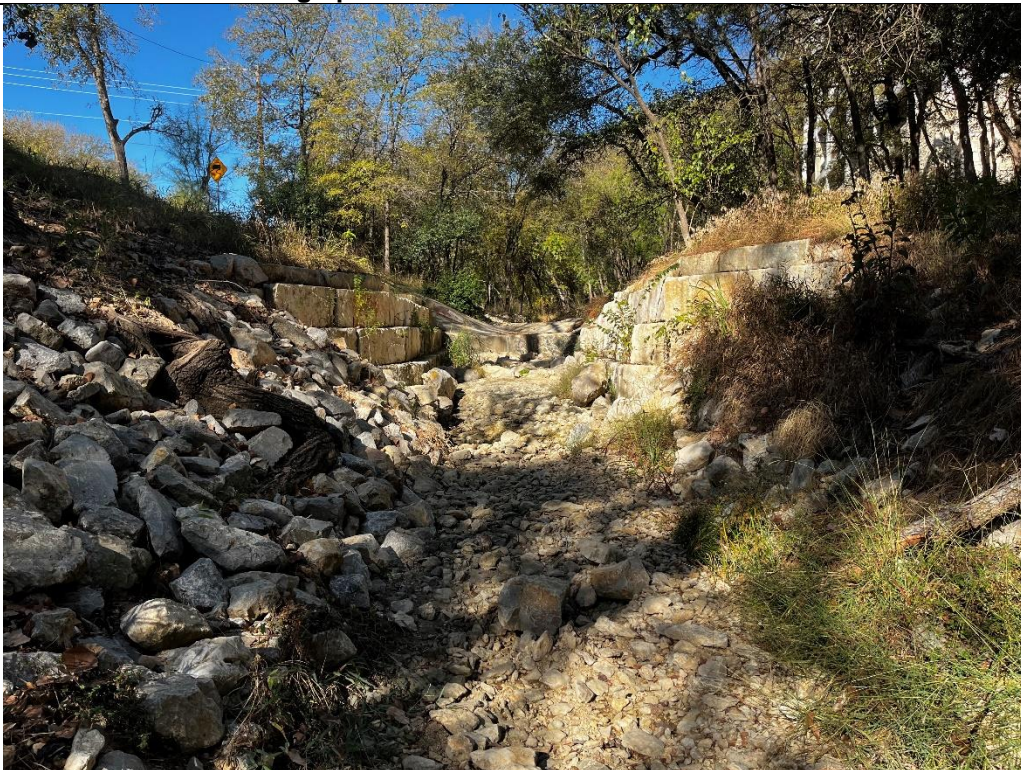
Photo 2. Station 2, directly downstream of gully control #1 and #2, facing upstream. Photo taken 11/21/2024.
