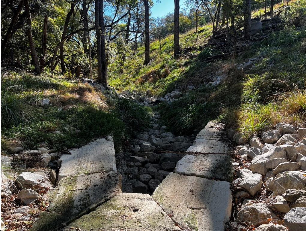
Photo 7. Station 7, facing downstream from grade control structure #5. Photo taken 11/21/2024.
