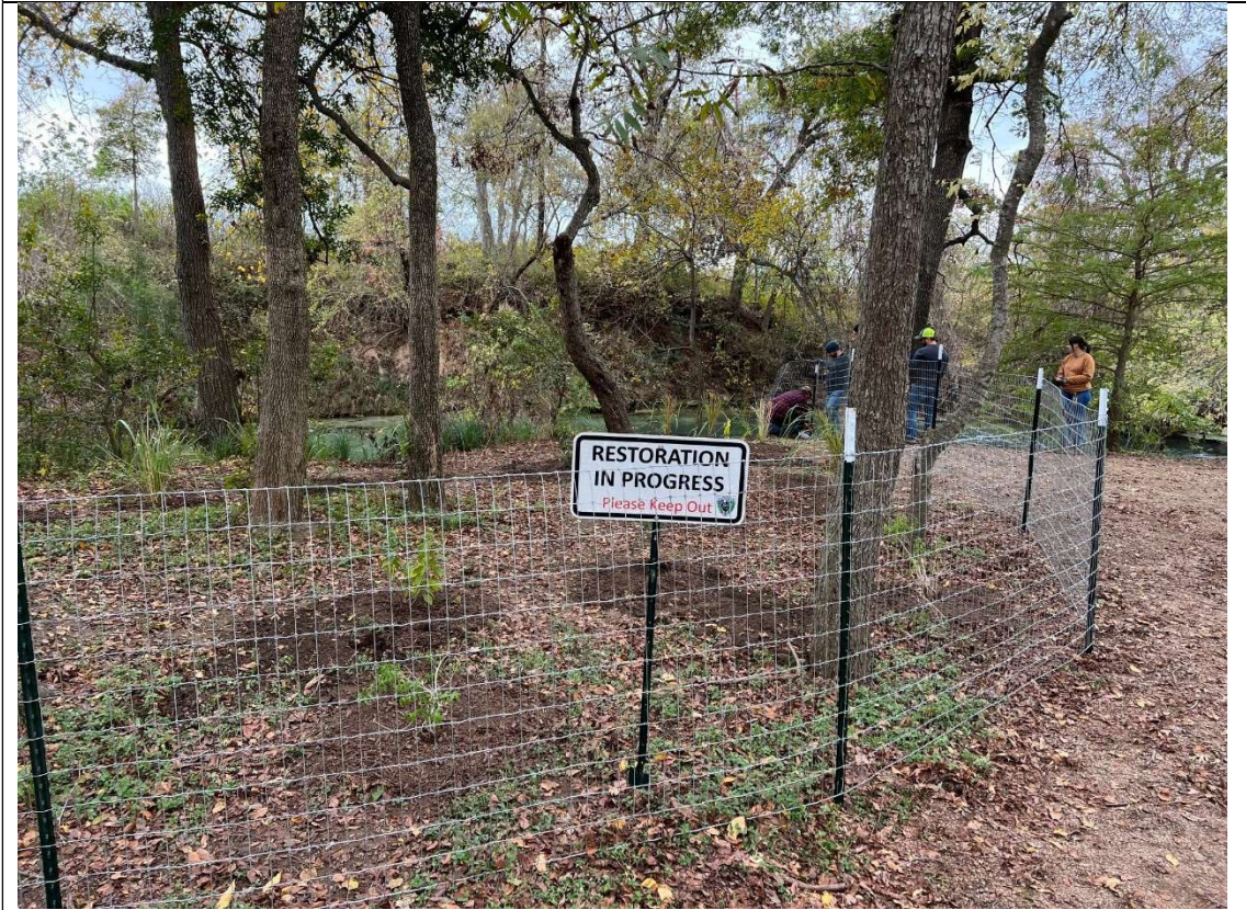
Figure 3. Native plantings and installed fencing to serve as a riparian protection zone, Crook Park/ Wildlife Annex.
