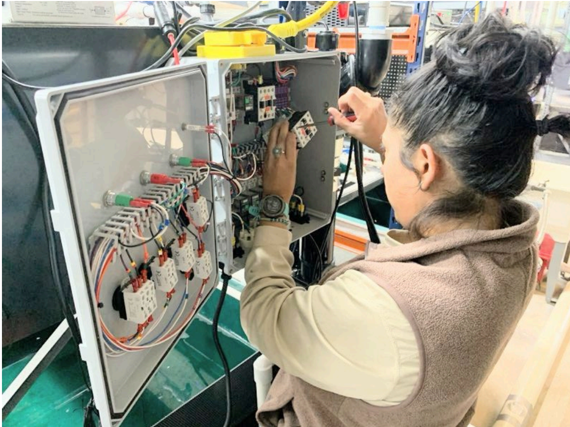
Figure 3. Dominique Alvear replacing a burnt circuit in the system controller box.
