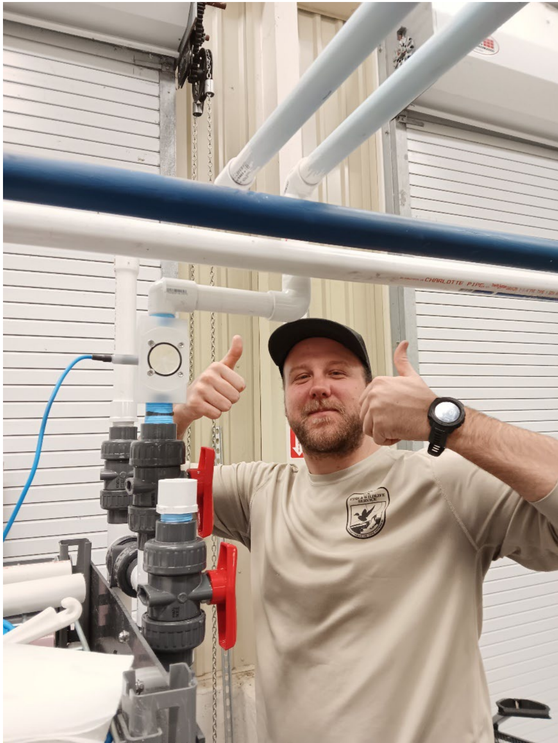
Figure 1. Jonathan Donahey finished plumbing the return line on quarantine rack 8.
