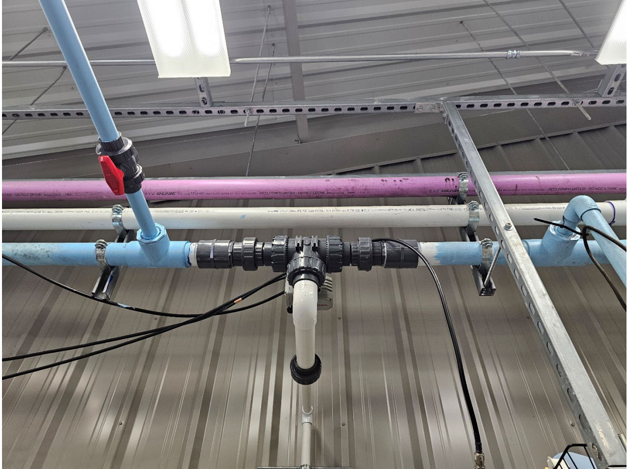
Figure 5. The completed supersaturation diversion project in the quarantine room at the SMARC.
