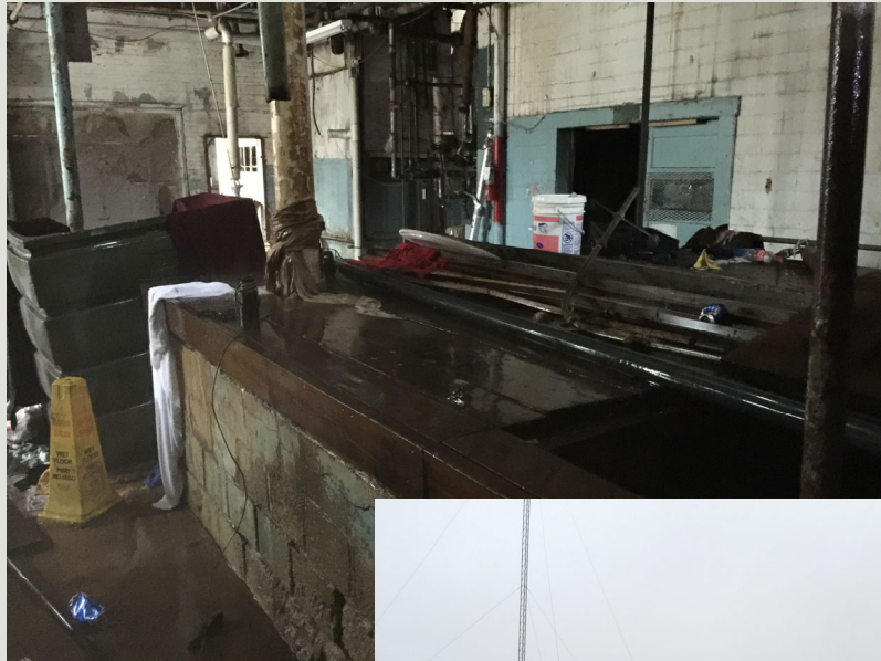
Abandoned well flowing inside building
