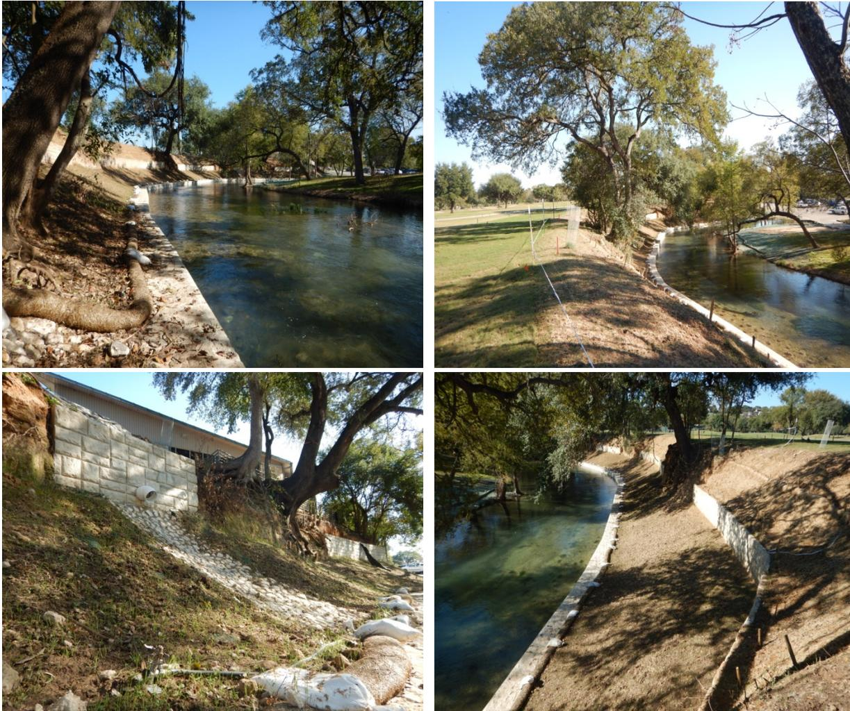
**Figure 3.2-12.** Photos of the bank stabilization work.
