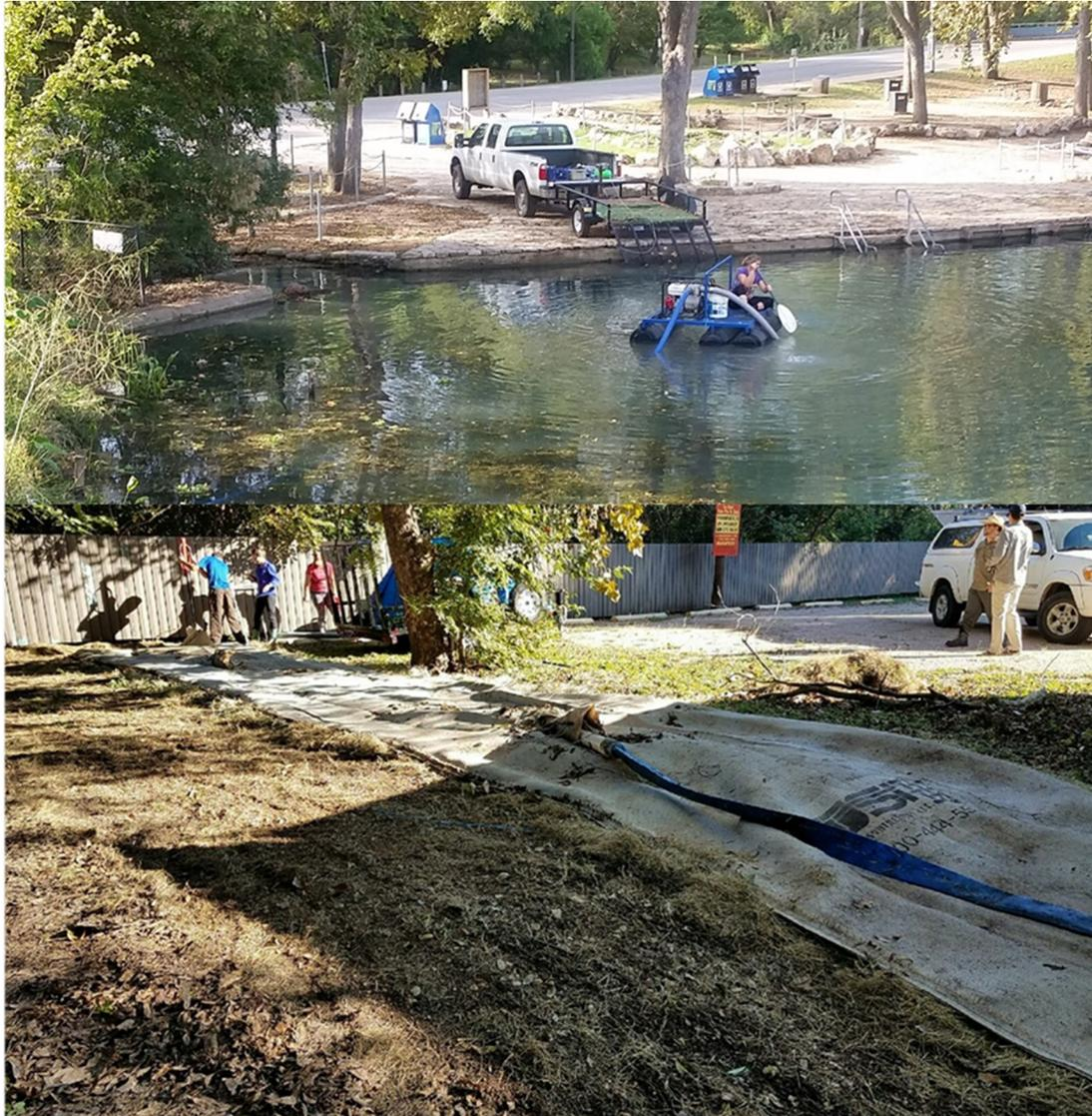
**Figure 3.3-19.** Arrangement for dredging at Rio Vista Dam (above) and placement of dewatering bag to minimize erosion and prevent turbid run-off back into river (below).
