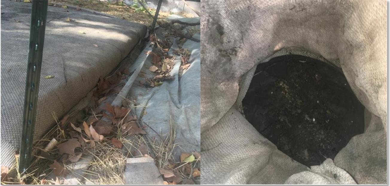
**Figure 3.3-20.** Accumulation of fine sediment in the dewatering bag (left) and type of sediment dredged (right) just upstream of Rio Vista Dam.
