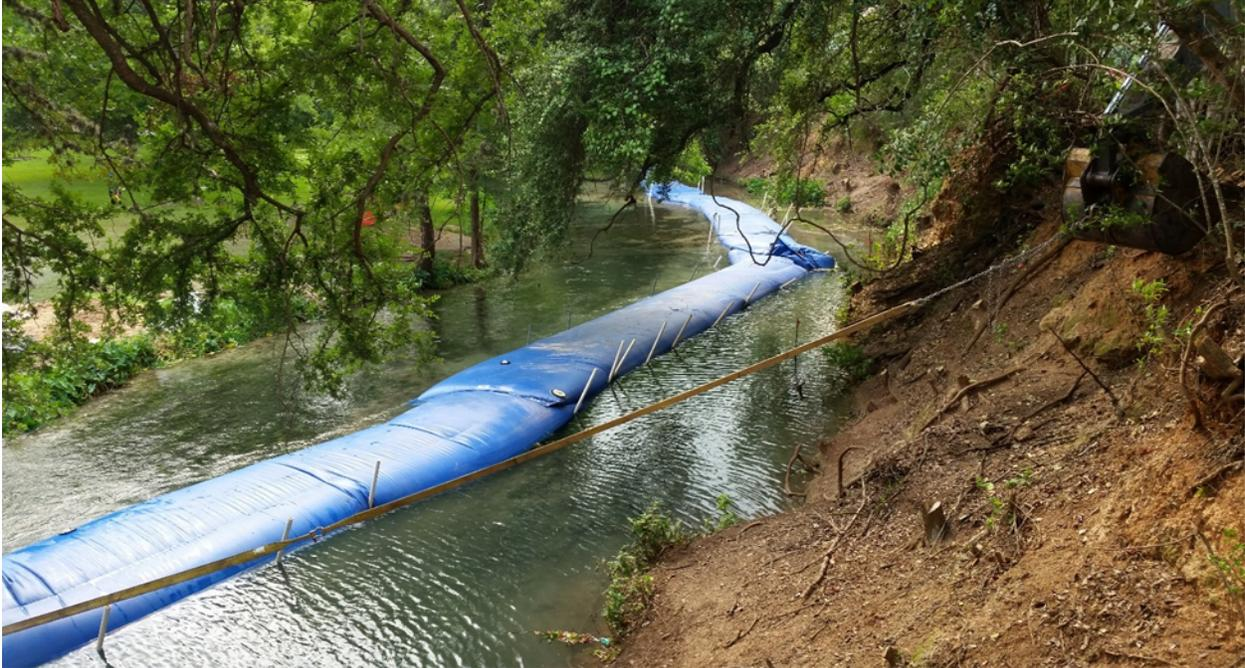
**Figure 3.2-11.** Water-filled bladder dams installed prior to project construction.
