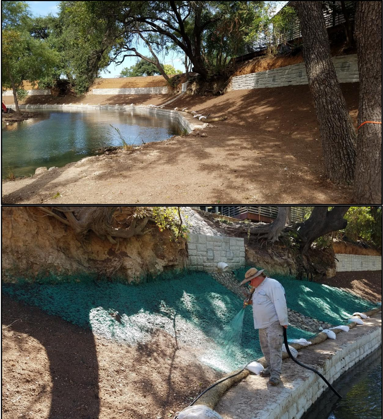
**Figure 3.2-15.** The completed bank stabilization work (top) and hydro-seeding process (bottom).
