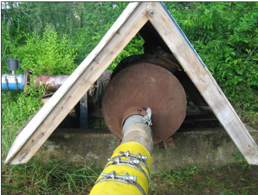
Figure 7. Wooden shade tent over in-line sampler at Aldridge 209 pump site.
