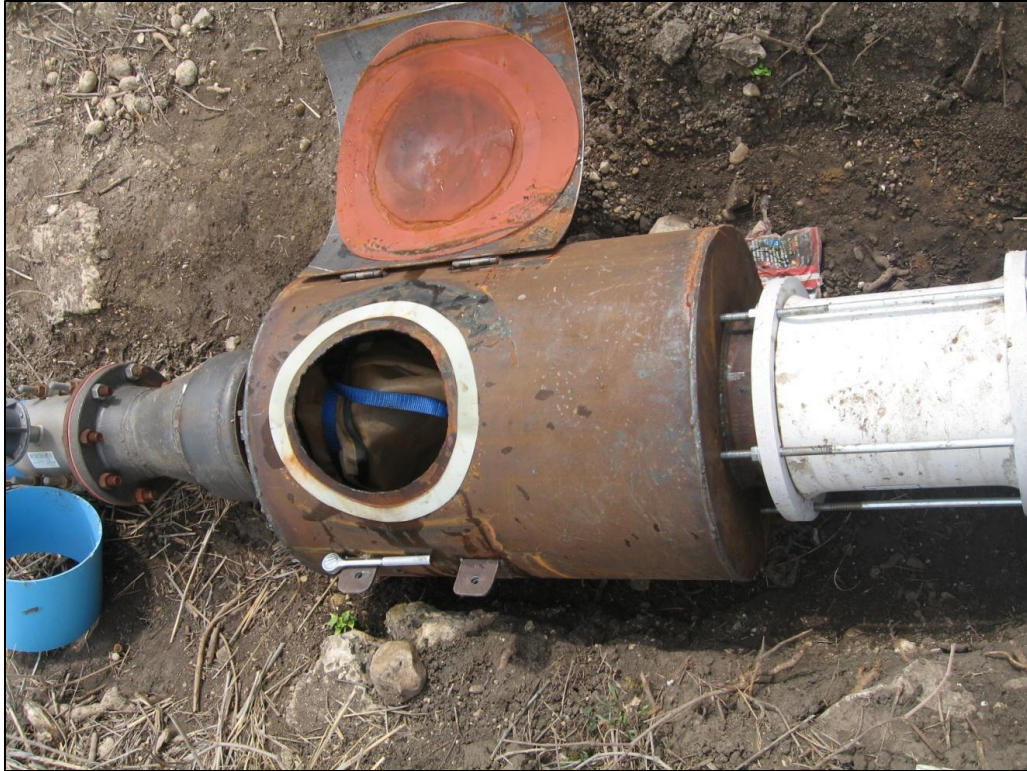
Figure 12. Net cinched inside of an in-line barrel sampler at the Tschirhart well.
