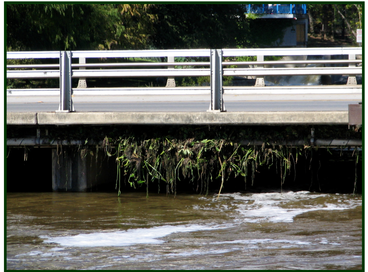
Figure 1. Photographs of (a) the City Park (Lion's Club) and (b) University Drive Bridge two days after the high-flow event in November 2004 (peak discharge unknown). The water is 12-18 inches above normal in the photos.
