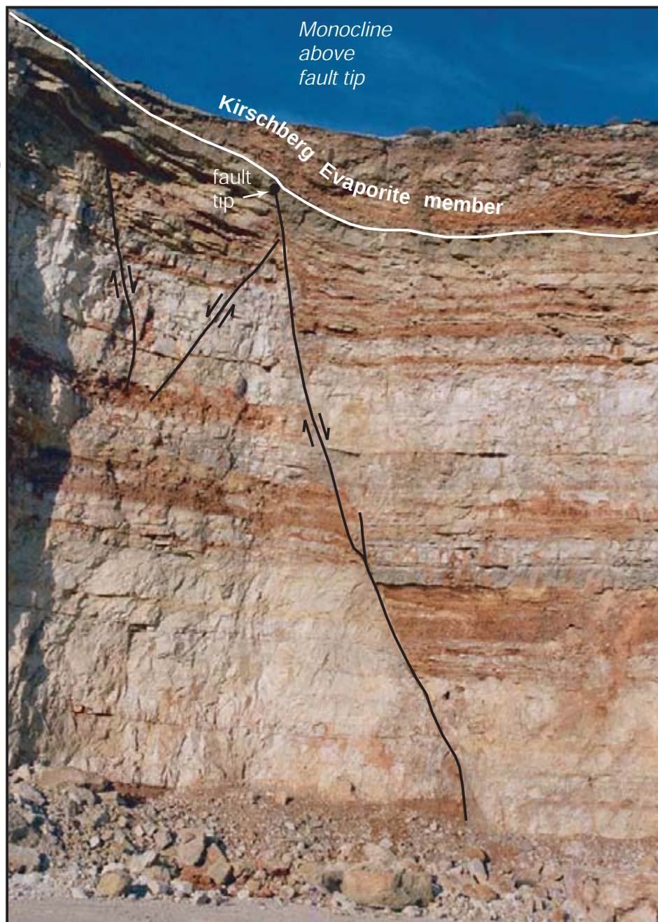
Figure 5-2. Fault in the dolomitic member of the Kainer Formation tips (terminates) upward into the Kirschberg Evaporite member. Displacement in the dolomitic member is replaced by monoclinal folding in the overlying Kirschberg Evaporite member. Photo from the Beckmann Quarry, San Antonio, Texas. View is to the ENE, along the direction of strike of the fault.
