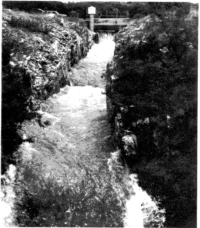
Water from June rains flow at record rates through the 10 feet wide by 15 feet high excavated channel from Seco Creek into the large sinkhole which drops 150 feet recharging into the Edwards Aquifer. Road crossing and gauge house is in background.
