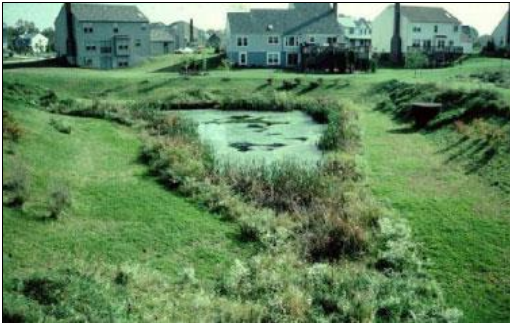
Figure 9. Extended detention pond to control erosive flows - pond empties within 2 days
