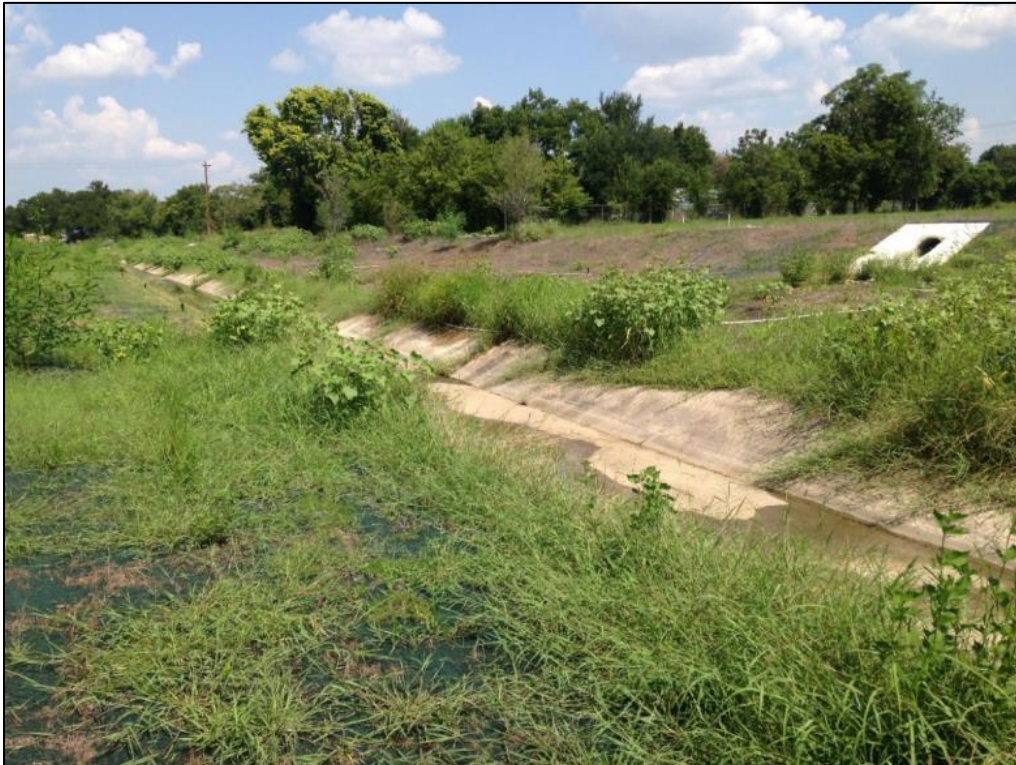
Figure A2. Willow Springs Creek near Senior Activity Center
