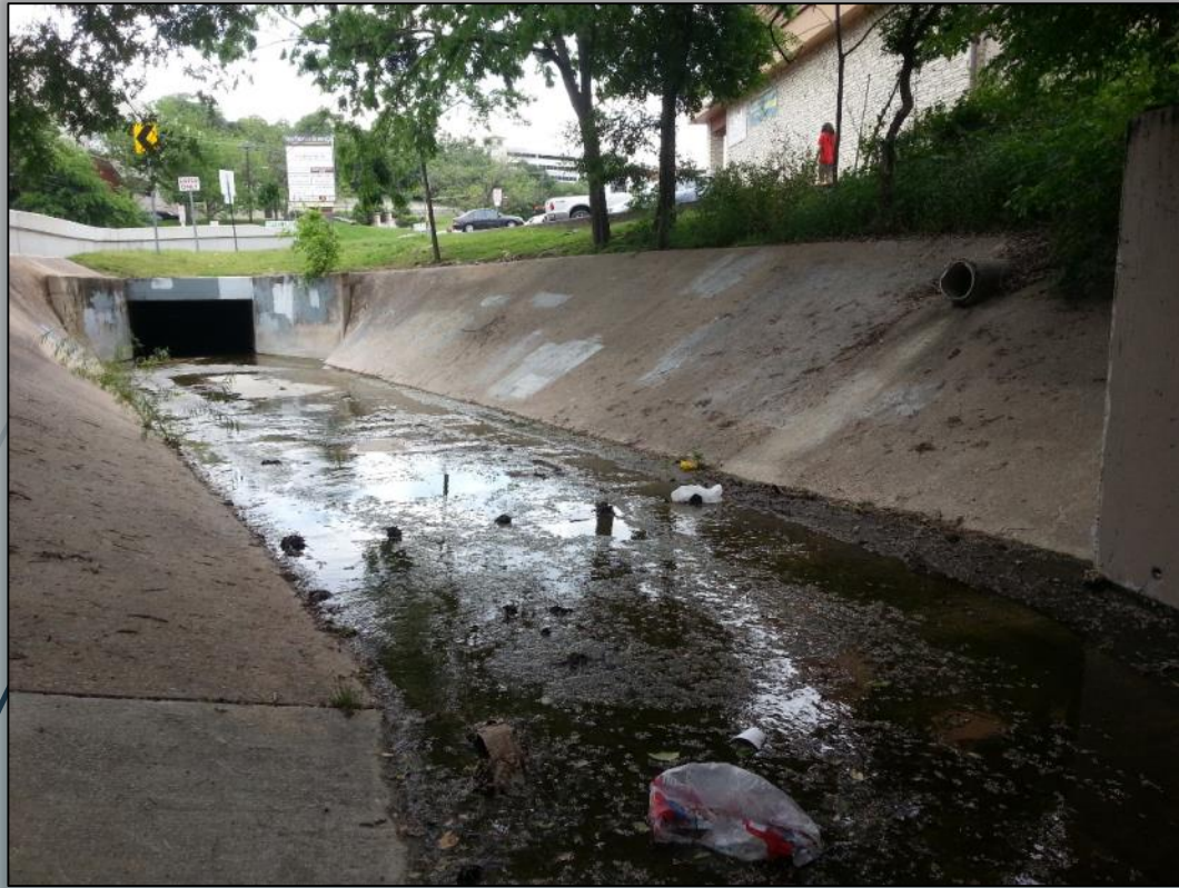
Concrete channel in Reach 1 – Downstream of Reach 2
