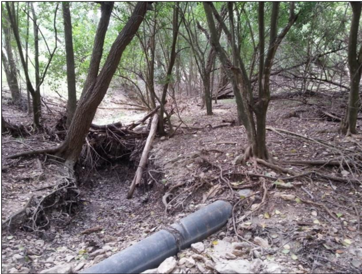
Figure 3. Sessom Creek stream erosion
