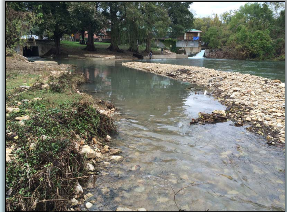
AFTER OCTOBER 2015 FLOOD
