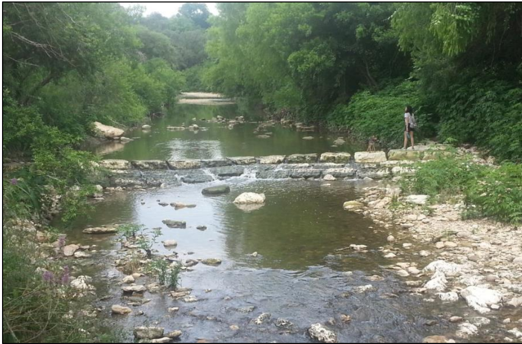
Figure 8. Grade control for stream restoration project on Shoal Creek in Austin, Texas
