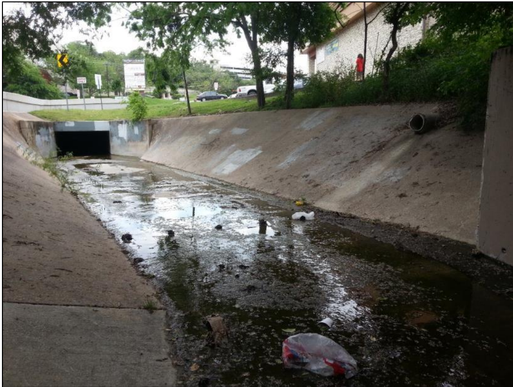
Figure C9. Concrete channel in Reach 1 – Downstream of Reach 2
