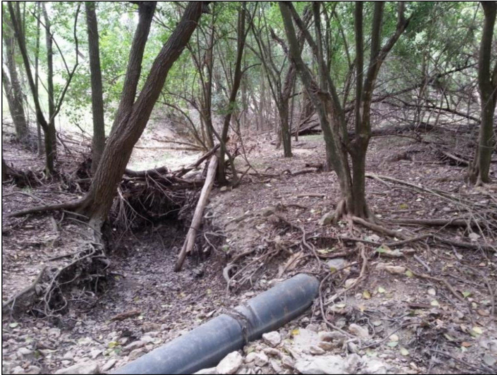
Figure A1. Sessom Creek stream erosion
