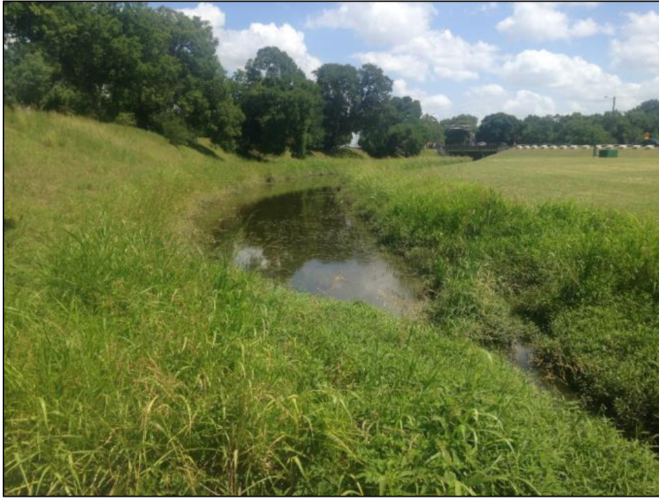
Figure A7. Purgatory Creek above Comal Street near confluence with San Marcos River
