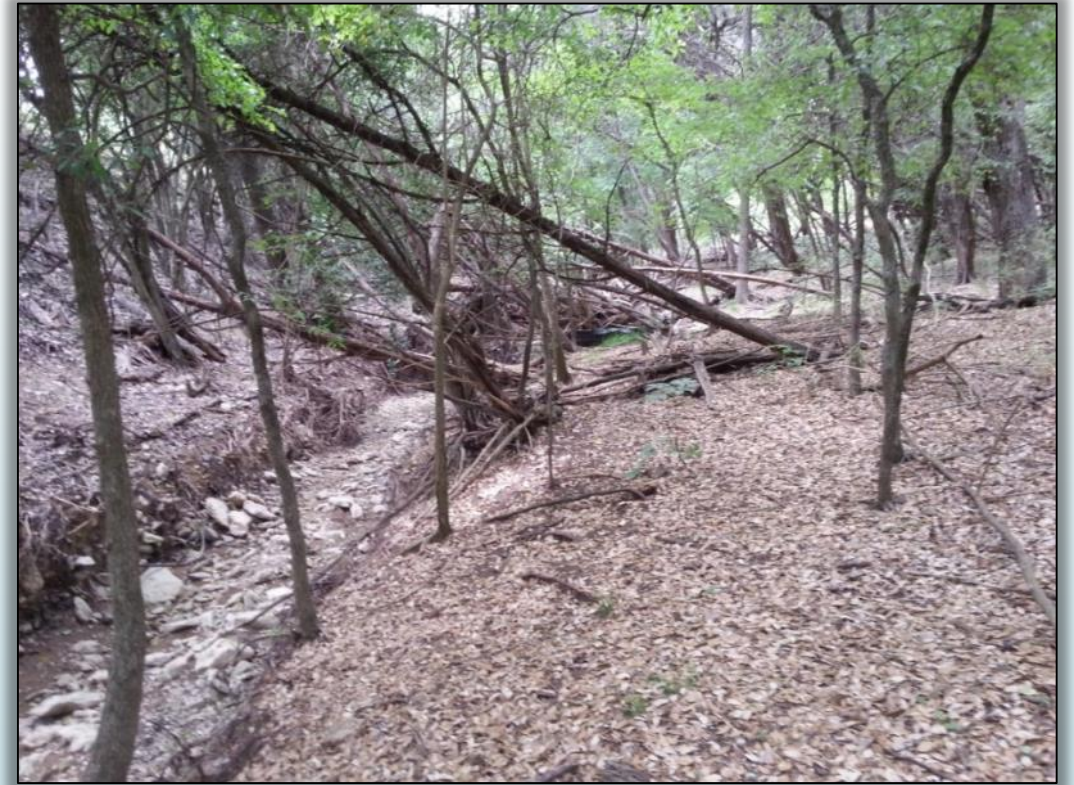
Reach 2 below Windmill Tributary – eroding streambank with poor riparian condition
