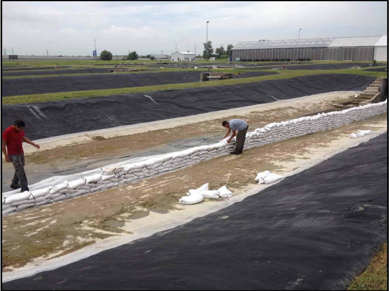
**Figure 12.** Sandbag wall being constructed to reduce the area of the experimental pond, thereby increasing water exchange rates to facilitate improved water temperature control.
