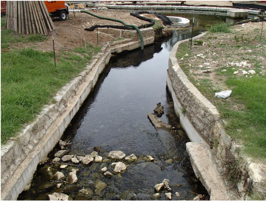
Figure 4: Surface flow throughout Spring Run 2.
