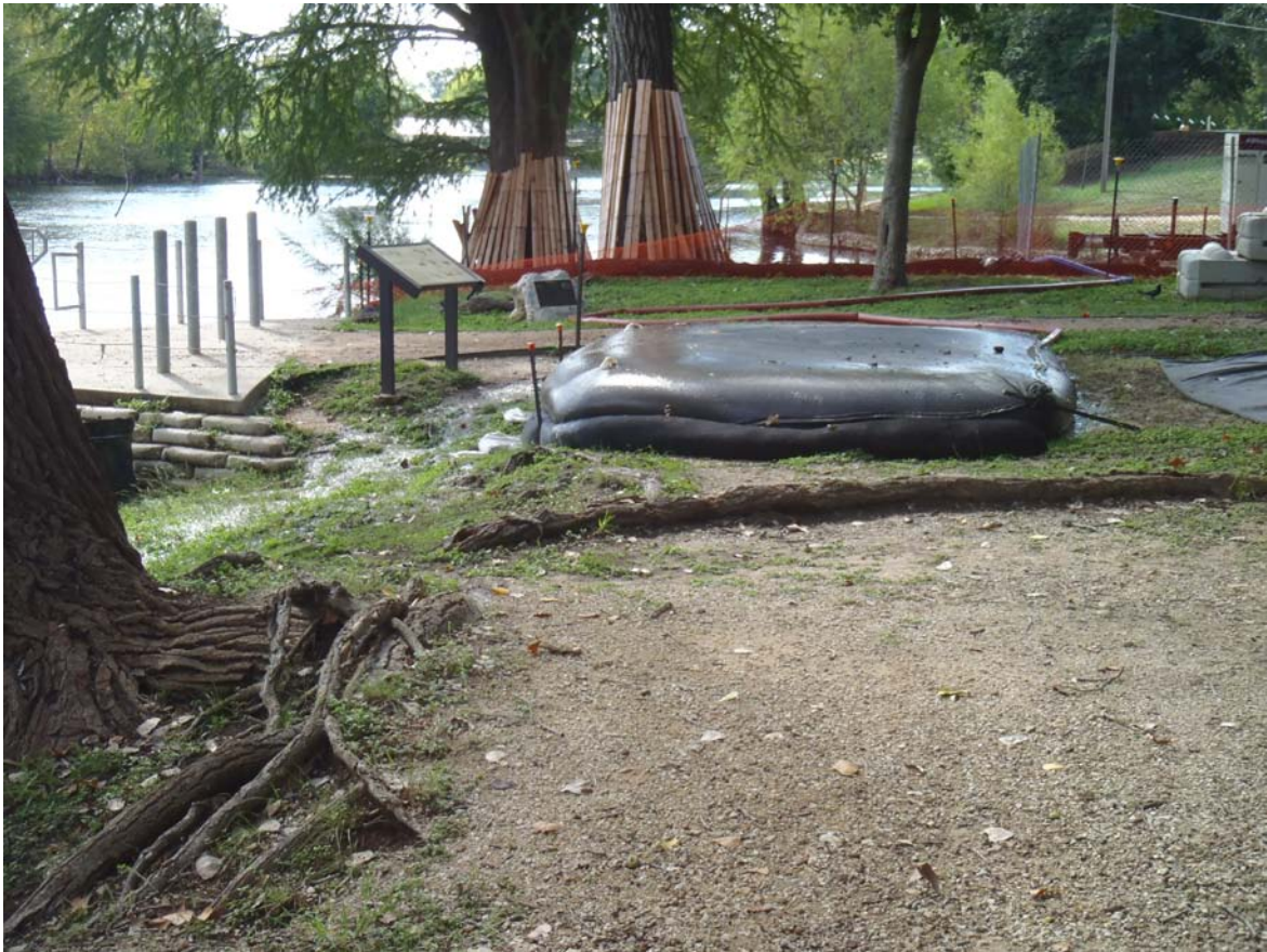
Figure 7: Siltation bag associated with the Landa Lake walls construction project.
