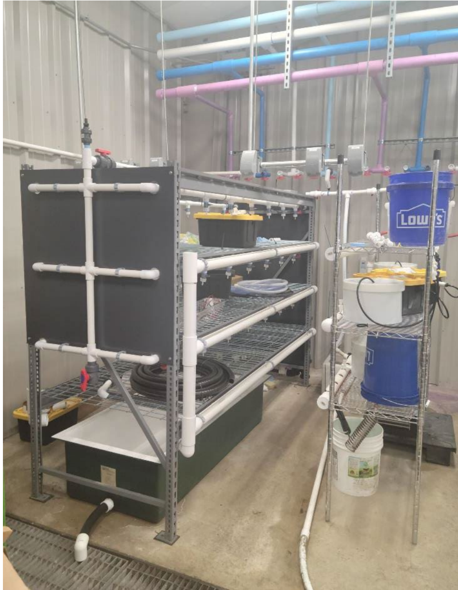
Figure 2. Construction of the new invertebrate rack system (left) in the refugia at the SMARC. Photo credit: USFWS
