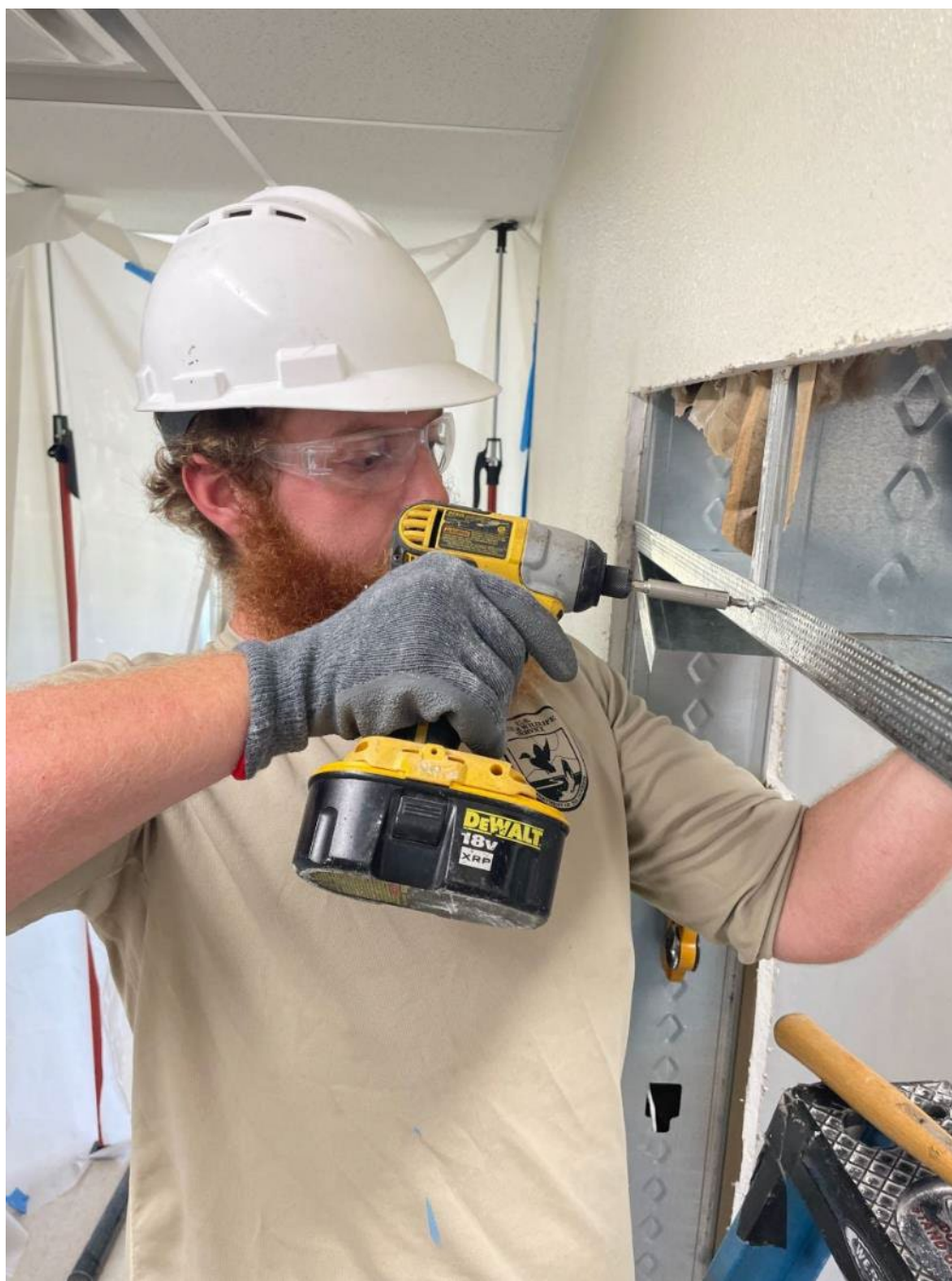
Figure 8. Braden West constructing the frame for the new office entrance. Photo credit: USFWS
