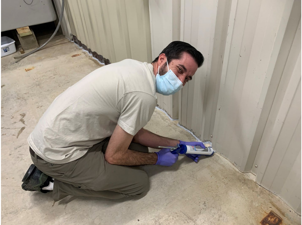
Figure 3. Adam Daw caulking the wall in the invertebrate room at the UNFH in Uvalde, Texas. Photo credit: USFWS
