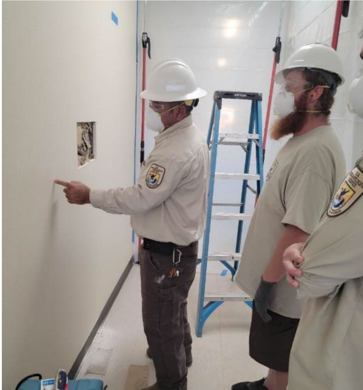
Figure 7. Modifications to the EARP building begin. Juan Martinez (SMARC) instructing Braden West and Tommy Funk on how to properly create a doorway in a wall. Photo credit: USFWS
