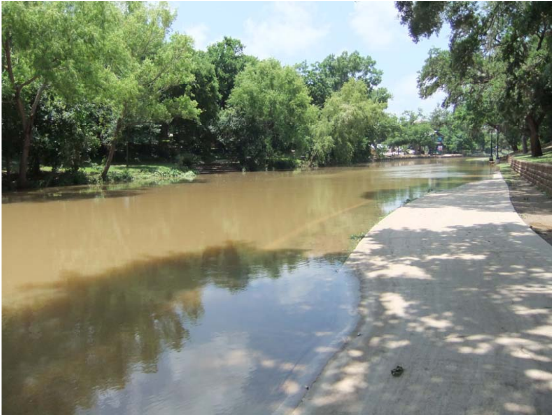
Figure 8. Flooding at the New Channel Reach, June 2010.
