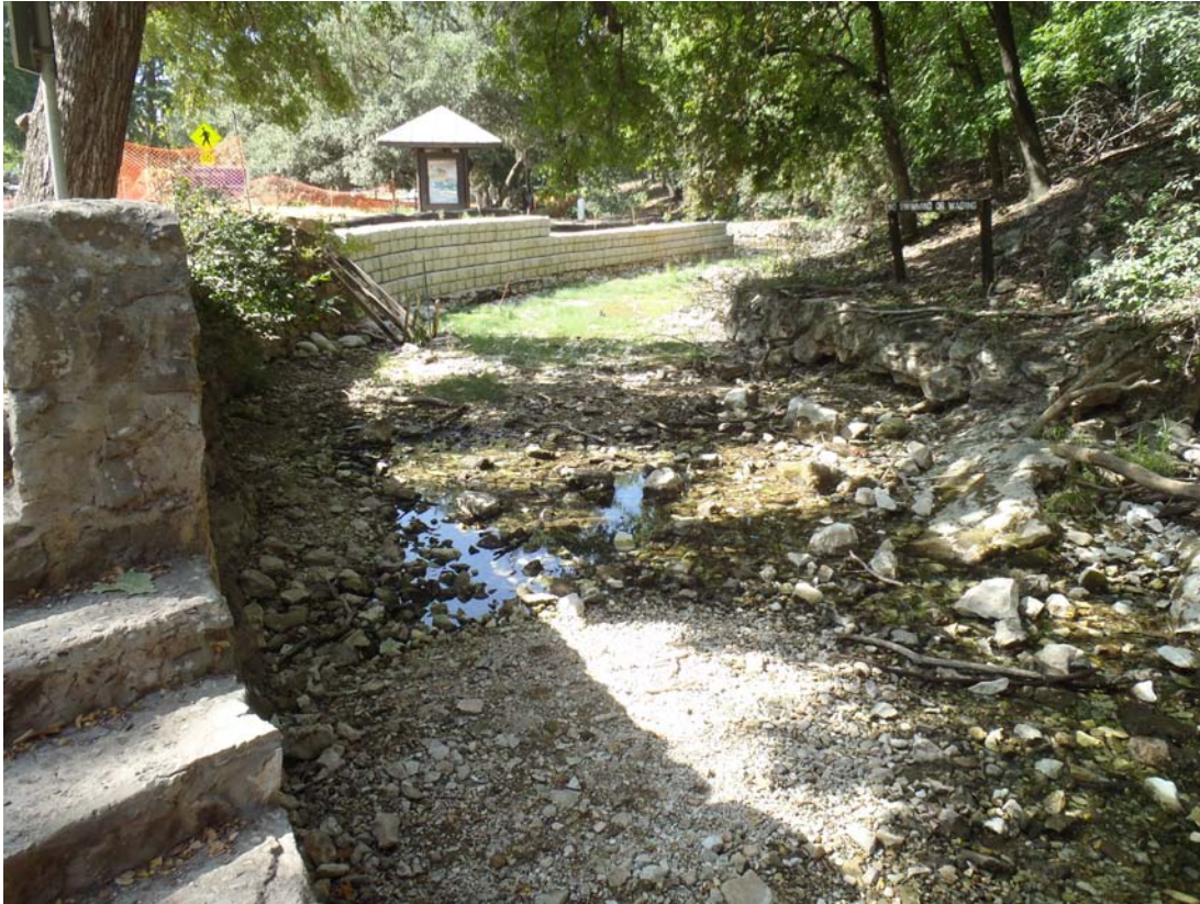
Figure 2: Spring Run 1 main channel looking downstream from main orifices).
