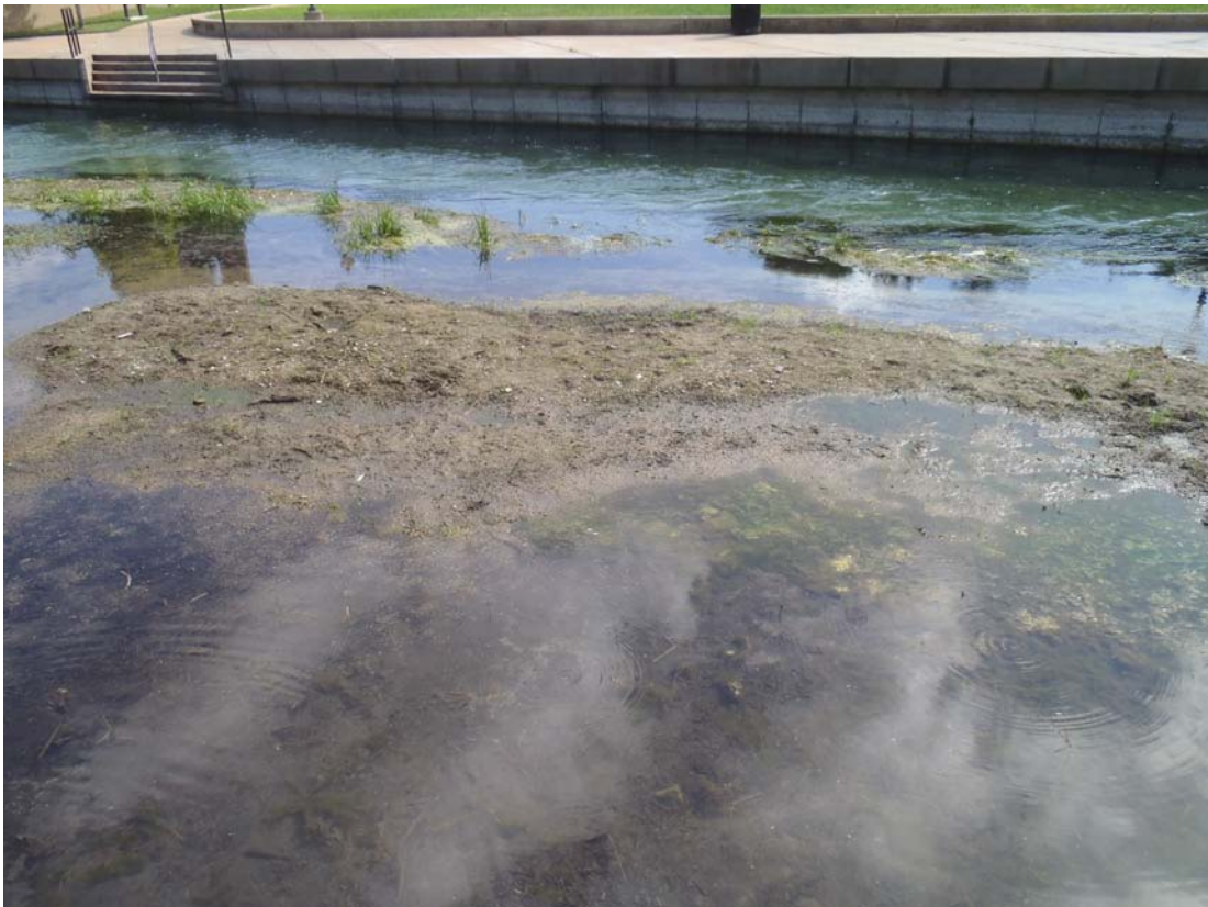
Figure 24: Exposed sediment in Sewell Park
